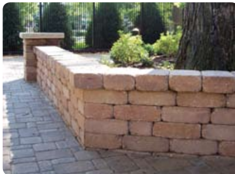
LedgeStone Retaining Wall
