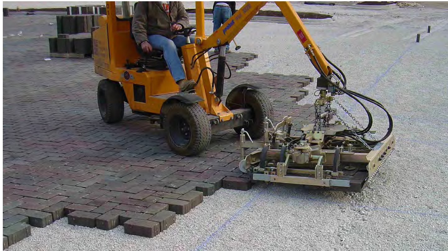
Figure 5. Mechanical installation of concrete paving units for PICP.
